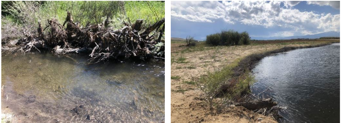
Figure 2. Example Log Structure streambank treatments. The larger wood in the bottom half of the right photo shows a Log Structure installed in Phase 3A of the CFROU. The left photo is an example Log Structure treatment from a project not on the Clark Fork River.
